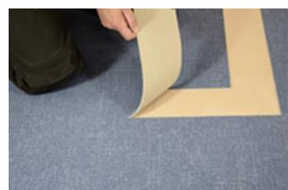
Apply a fresh layer of acrylic adhesive. Lay the Artline border into the adhesive and using a rubbing board press the border firmly into the adhesive (see below).
