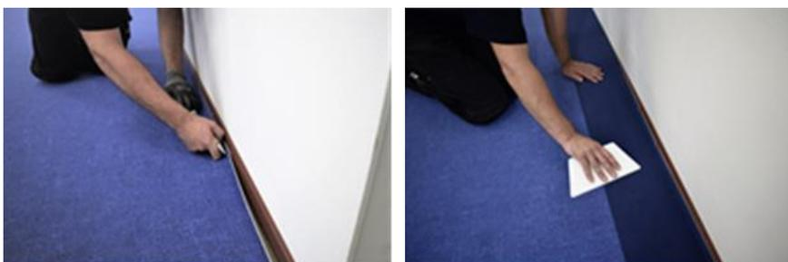
Remove fresh adhesive residue immediately with a clean white damp cloth.
