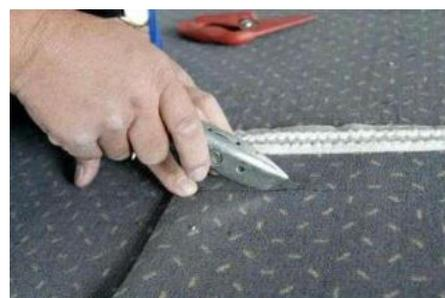
If this is not possible because the pattern does not proceed parallel to the seam channel, the pattern and the print edge must be cut with a rolling steel rule and a sharp hook blade.
